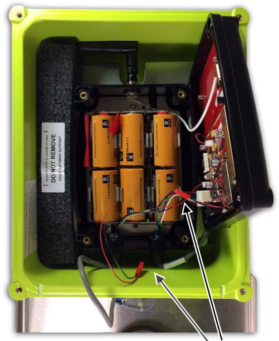
XT-Series battery cable disconnected during battery installation
